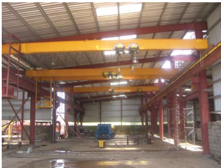
Partial View of the Plant
