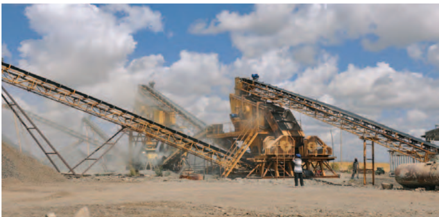
The newly erected aggregate crushing plant in operation at Bole-Belo
