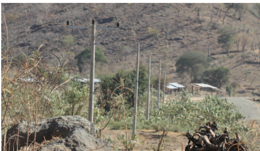
Erected SABA's concrete poles in Sanja, Gonder
