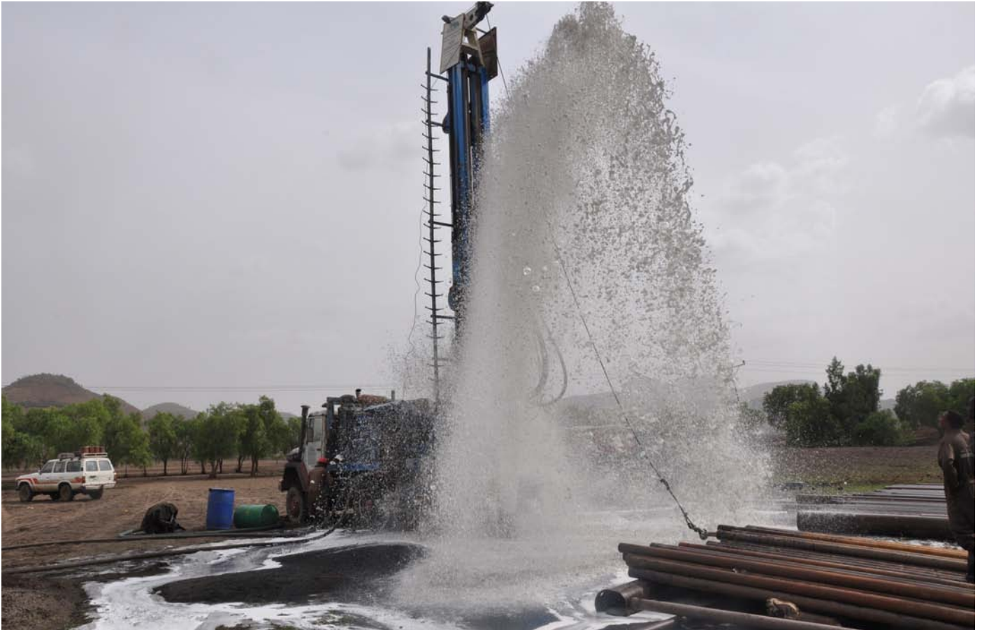
The drilling rig developing the well at Gohala town Eastern Belesa Woreda, Northern Gonder Zone
