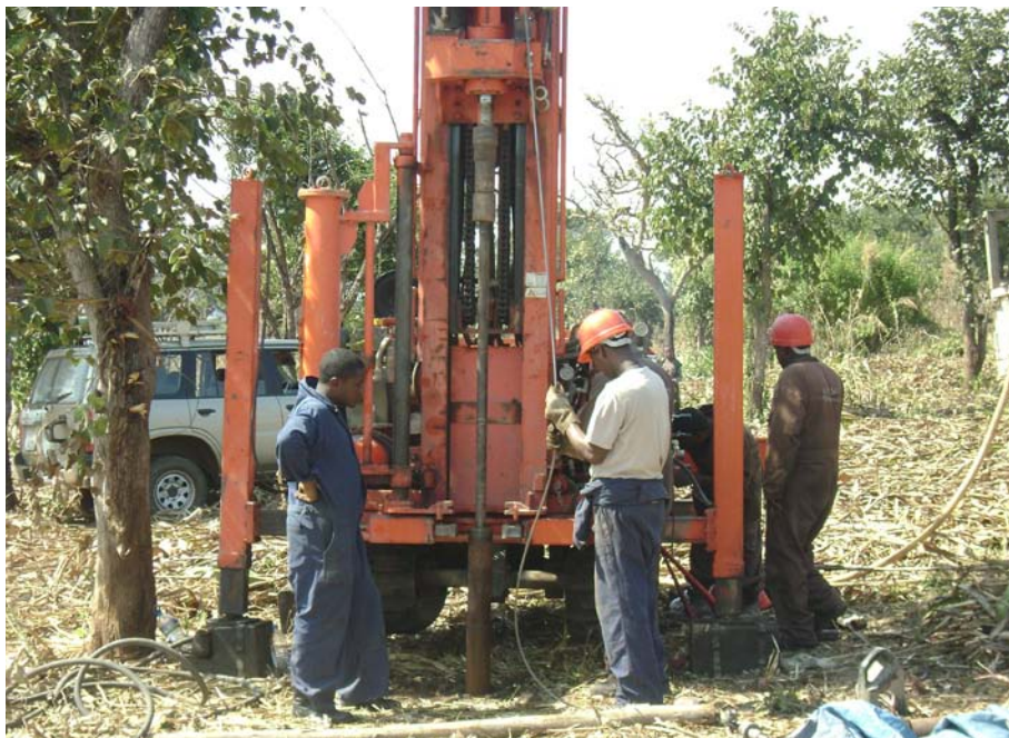
Drilling on progress at the dam site
