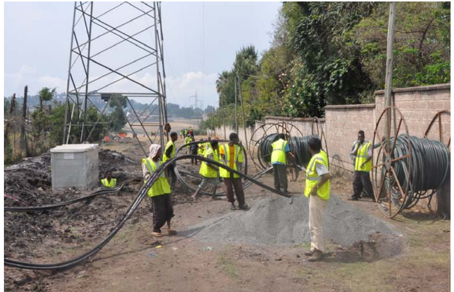
Underground cable installation in one of the sites around Kaliti
