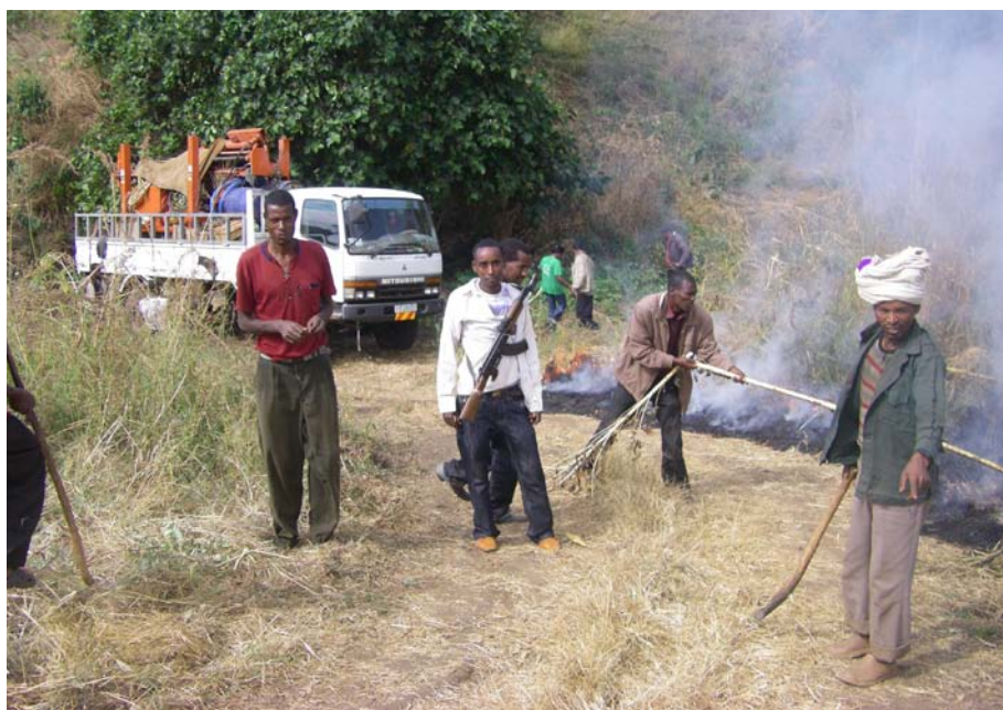
Rehabilitation of the earth road leading to the dam site
